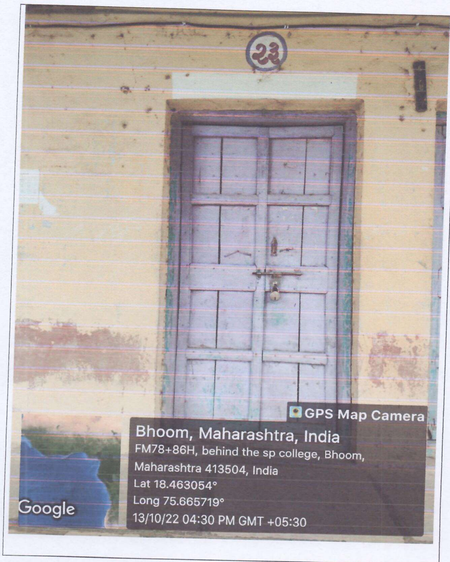
PHOTO NO. 58 HALL NO. 23 STORE ROOM
